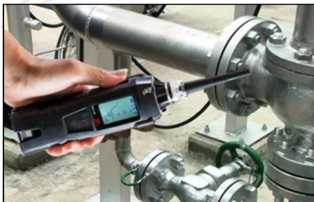
For gas pipe joint
